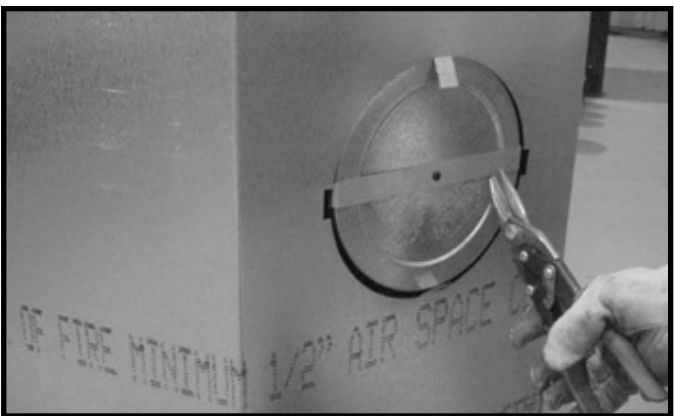
Figure 6.7 (Generic Fireplace Shown) Cut the metal retaining band and fold the sides out.
