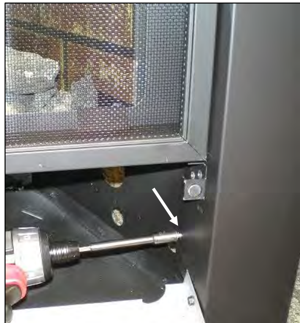
Step 4: Open Lower Panel and install screws through surround. Raise Lower Panel and replace screws.
