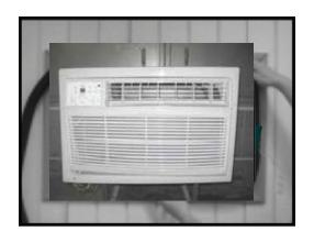
1. Install the 1" x 1½" x 84" long stuffer-seal between the wall-sleeve and the unit. A flat-bladed screwdriver or putty knife is recommended.
