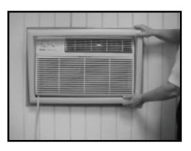
3. Pull cord through trim frame, then slide in unit until flush with wall.
