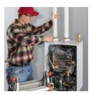
1/2" gas connections (subject to local code) and 2" PVC venting help reduce installation time.
