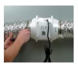
Attach the ducts with clamps.
