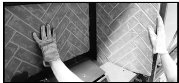
Figure 11.3 Install Side Refractory Panel (Right Side Shown)
