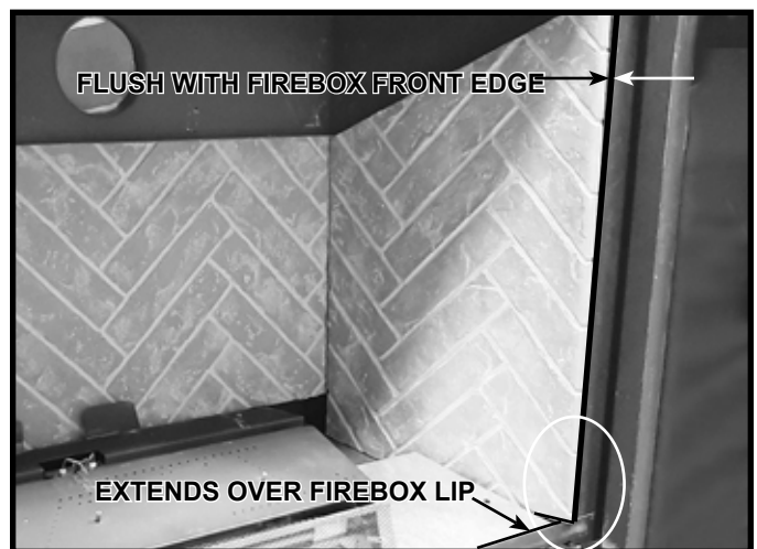
Figure 11.4 Side Refractory Panel Installed (Right Side Shown)
