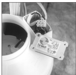
Romex wiring – Top View
