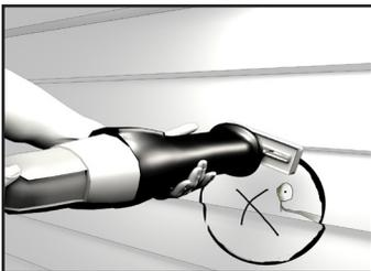
**1** Using the duct connection of the outside hood, outline the intake & exhaust holes to be cut. The holes should be slightly larger than the duct connection to allow for the thickness of the insulated flexible duct. Cut a hole for both the intake and exhaust hoods.
