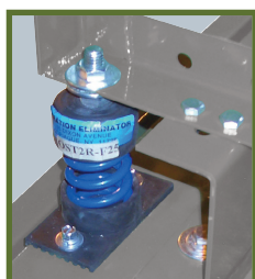
9200-VIB SERIES With Internal Spring Vibration Isolation
