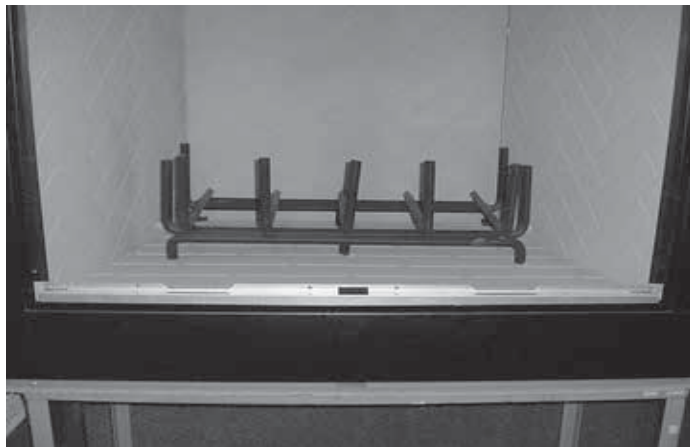
Figure 2 - Installed Door Track
