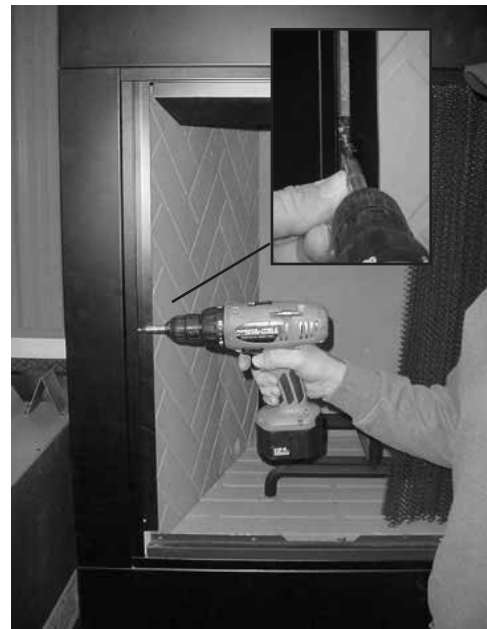
Figure 5 - Fastening the Side Filler
