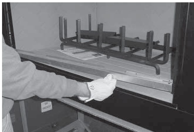
Figure 1 - Install the Door Track
