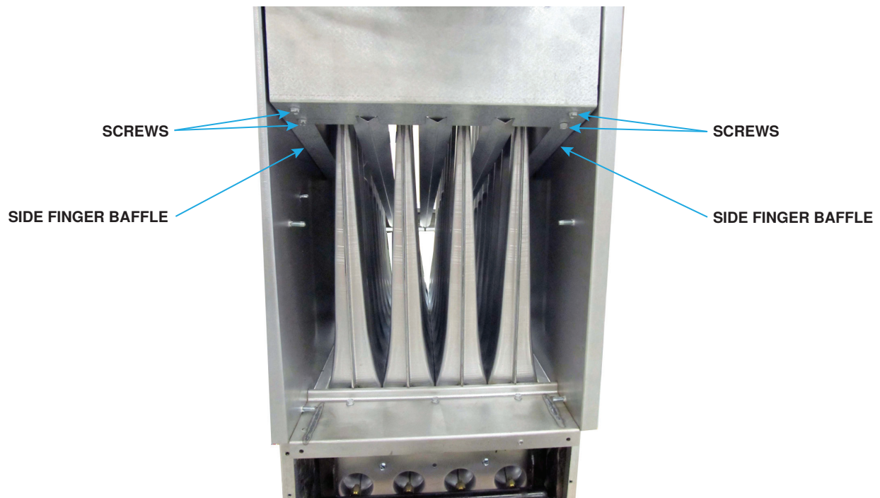
Figure 4. Side Finger Baffle Removal
