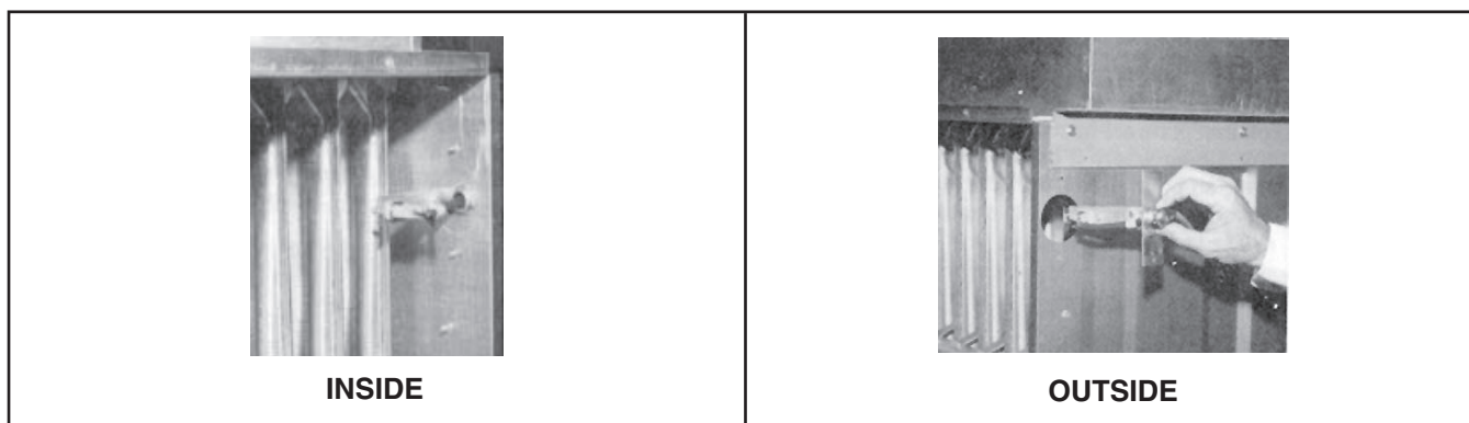
Figure 27. Limit Switch Access
