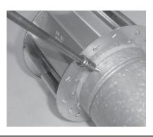
STEP 7: Place continual 1/4-inch bead of silicone sealant around circumference of venter outlet collar.
