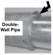
STEP 3: Drill three small holes spaced equally around double-wall pipe below sealant ring. Secure joint using 3/4-inchlong sheet metal screws. Do not overtighten screws.
