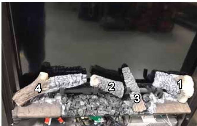
Figure 4.19 Log Identification
